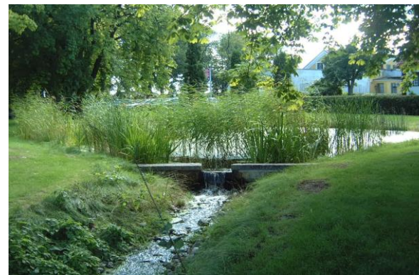
Constructed wetland (Self-purification)
