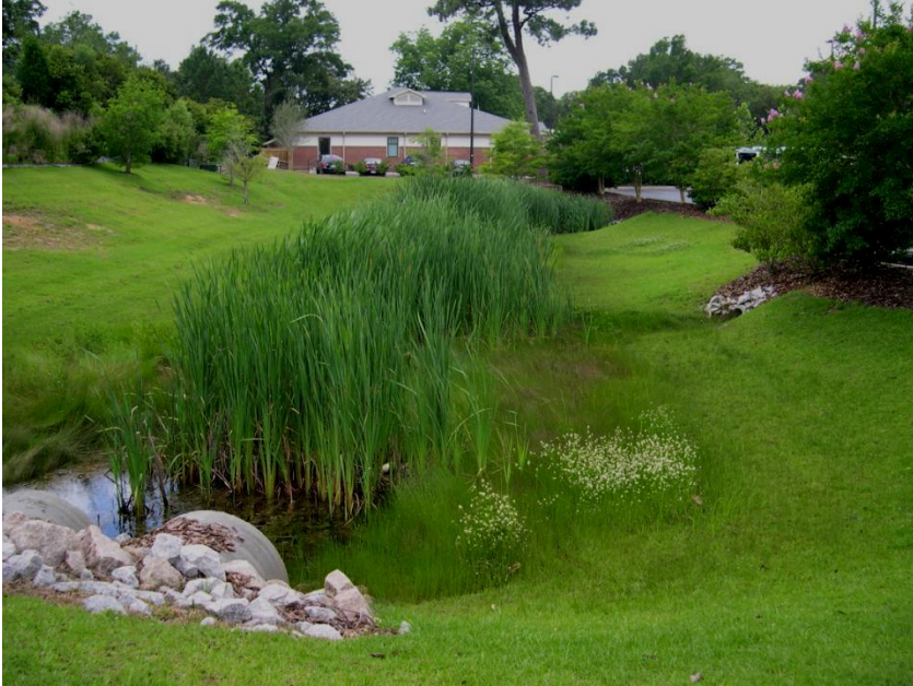
Urban stormwater runoff treatment (Charleston, USA)
