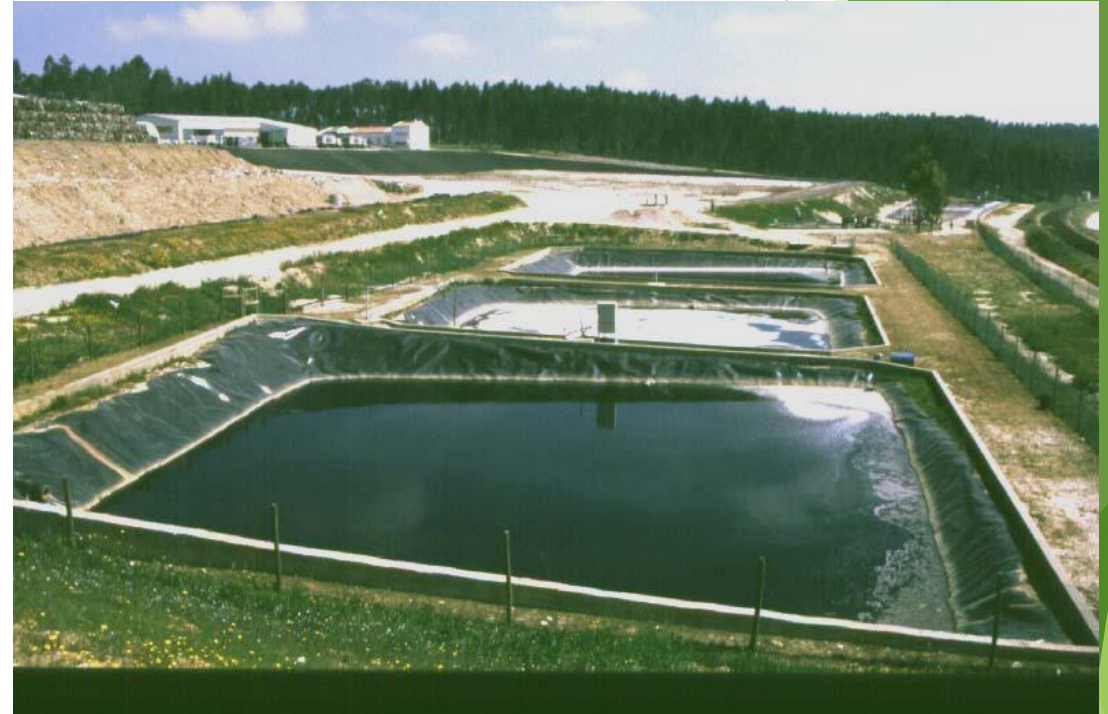
Landfill leachate treatment (Leiria, Portugal)
