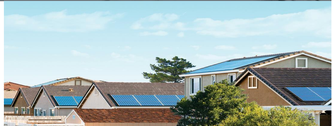
Solar Home Community, California
