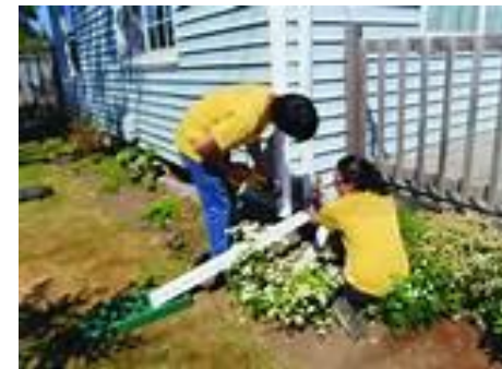
Roof disconnection / water butts
