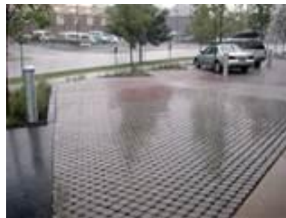
Road permeable pavements / SuDS
