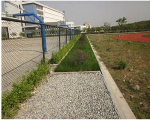
Bioretention Cell with Gravel Inlet Chamber
