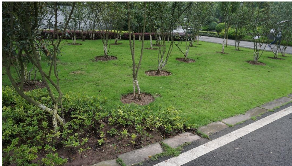
rainwater retention control technology on the side of the road
