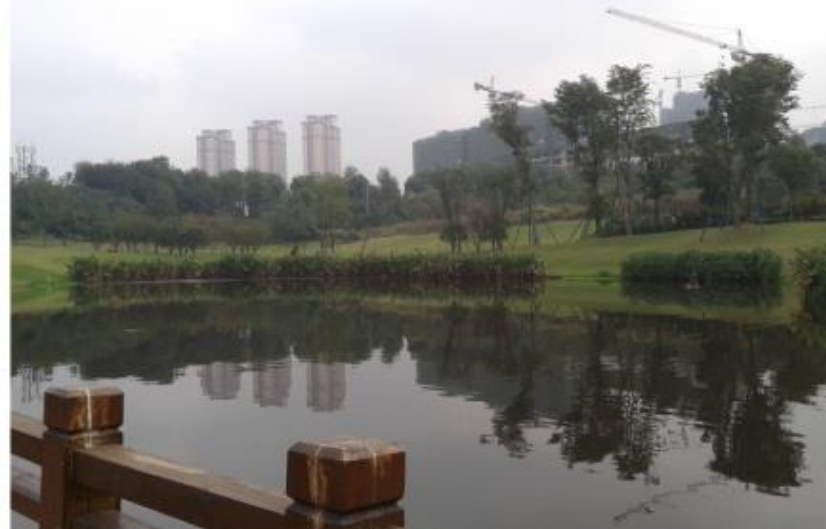
生态护岸 Ecological embankment
